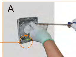
A Uninstall the mounting bracket from fixture base plate by unscrewing the 2 hex socket studs.
